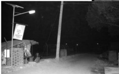
Solar street lighting by GAIL at Khanpur village at Pata, UP
