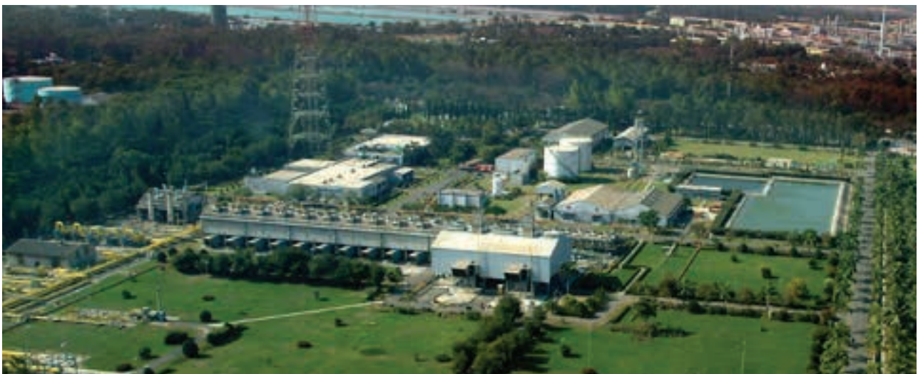
Aerial View of GAIL, Hazira
