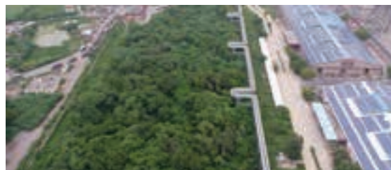
Extensive Green belt maintained at GAIL Pata plant along with Rooftop Solar PV plant at GAIL, Pata
