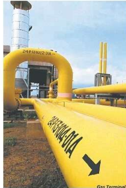
The company is building six gas pipeline projects spanning 6,800 km.
