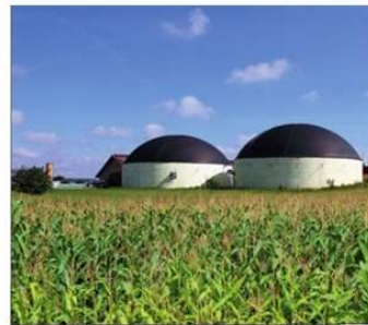
Clear the air with the domes
