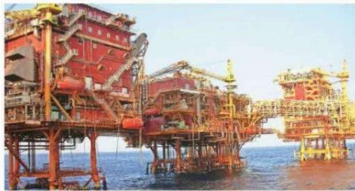
ONGC processing platform at the Mumbai High offshore oilfield. Wikimedia Commons
