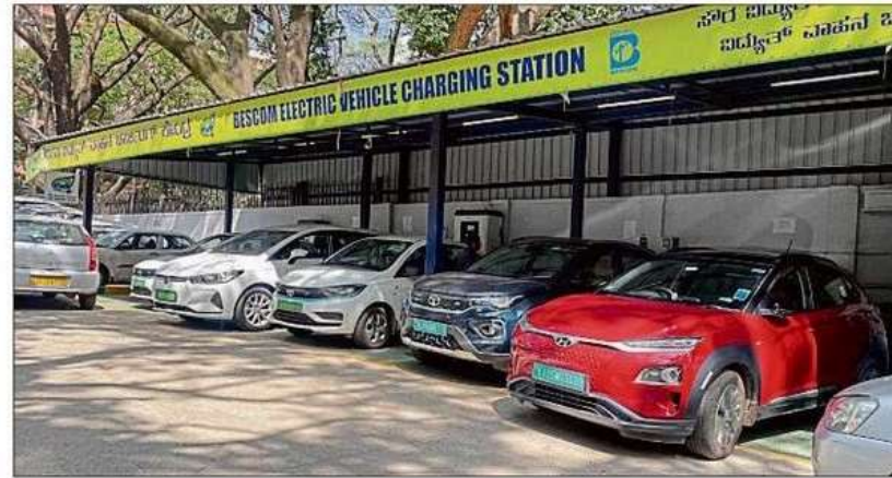
A Bescom charging station at KR Circle. DH FILE PHOTO
